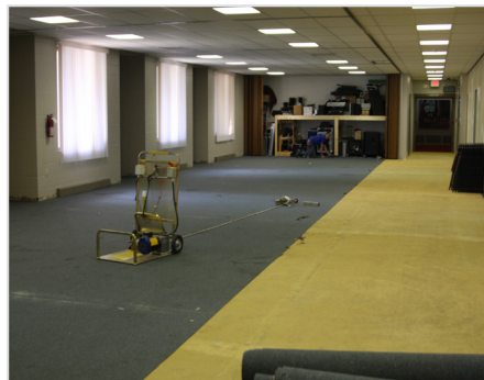
Carpet has been laid in the center wing.
